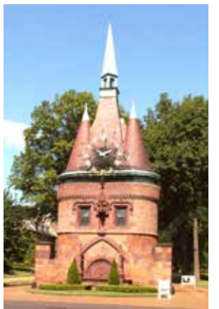
Washington Terrace Entrance
