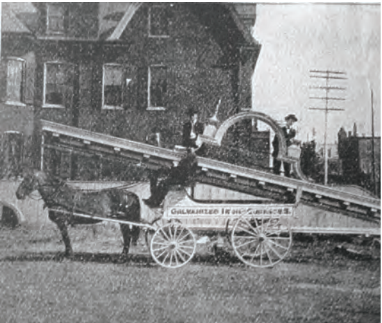
LEFT: Luepker Cornice delivery wagon transporting a complete cornice.
