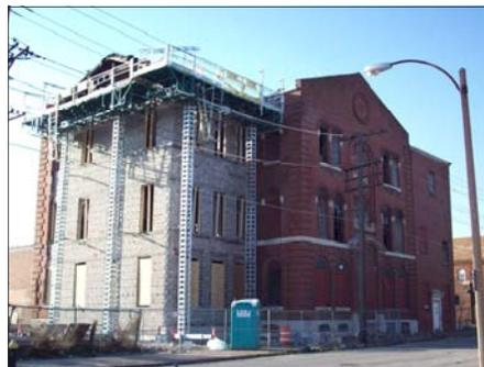
pany have framed up and closed off the massive opening along the north end of the building. This work follows the rebuilding of the entire south wall with concrete block, made possible by contributed services, supplies, equipment, and labor from several contractors affiliated with the Masonry Contractors Association and the Masonry Institute of
