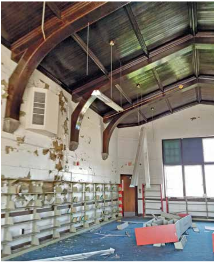
Hammerbeam construction in the auditorium
