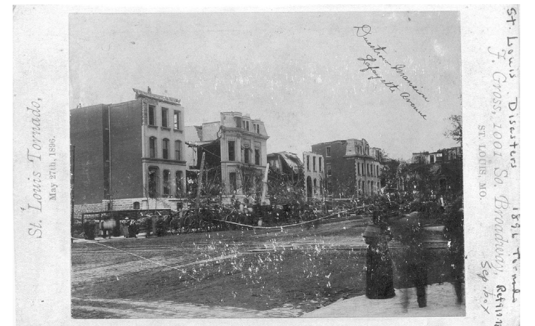
1896 Tornado Damage at Lafayette and Jefferson. Duestrow family home one of three damaged homes on the left, St. Louis Public Library.
