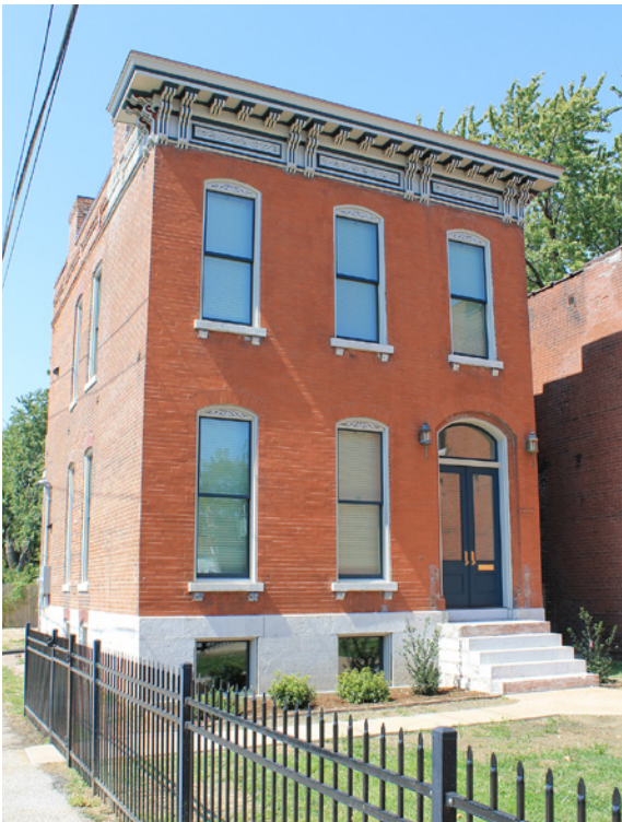
1211 Tower Grove Avenue, home of Oscar and Mary Waring 1884-1911
