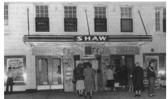
These photos show 3901 Shaw when it was the Shaw Theater (above) as well as before (top left) and after (top right) rehab.
