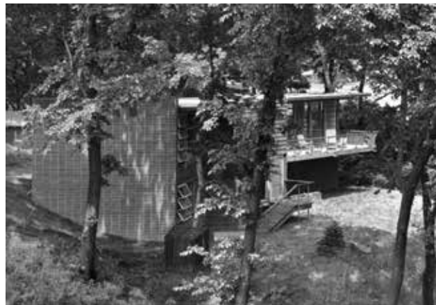
Farthing Residence, 8221 W. Main Street, Belleville, Ill
