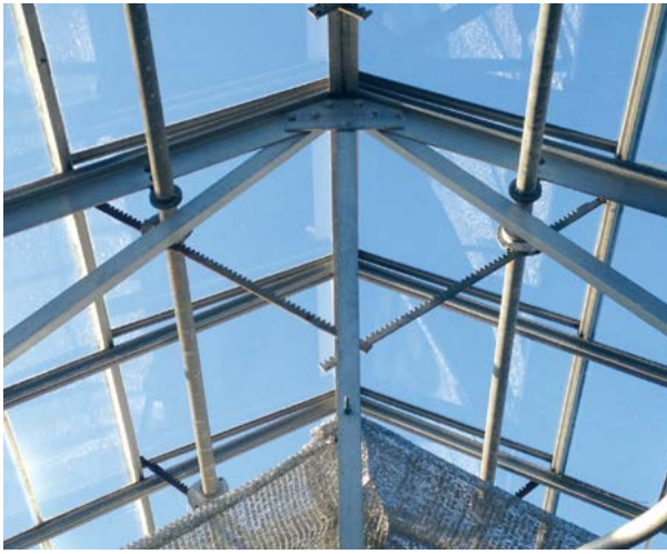
Structural detail of a greenhouse. Note the adjustable nets that filter sunlight.
