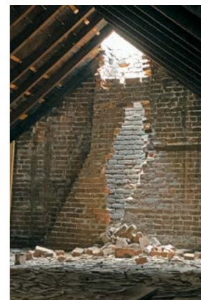
Chimney collapse
