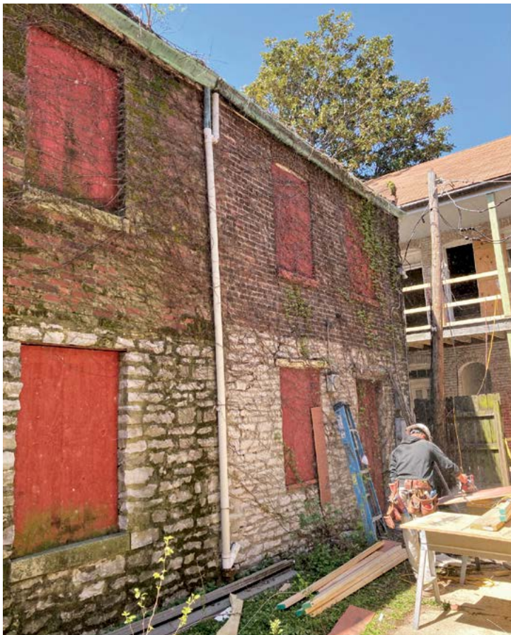
Rear "ell" portion of the front of the building with two types of stones
