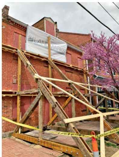
Brace supporting the primary façade.
