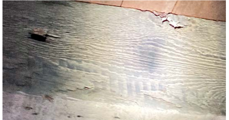
Vertical kerf marks of a reciprocating saw, and hand planed subfloor boards
