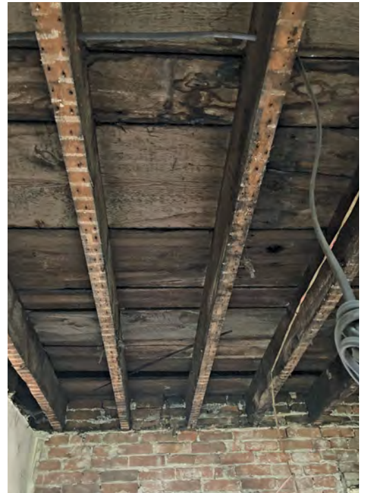
Old growth sub-floor boards up to 24" wide
